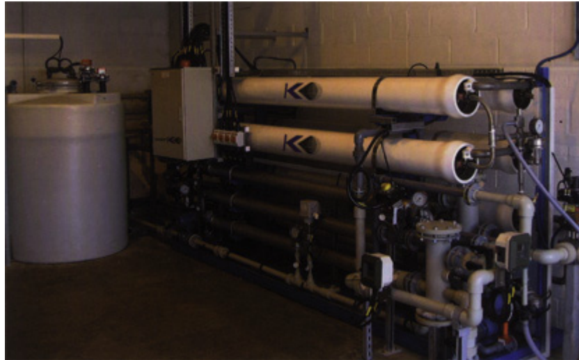
Typical RO Installation of a brine waste water
